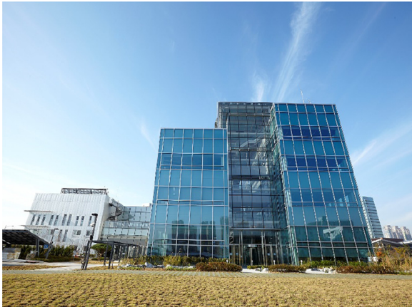
Fig. 4. Front View of Subject Building.
